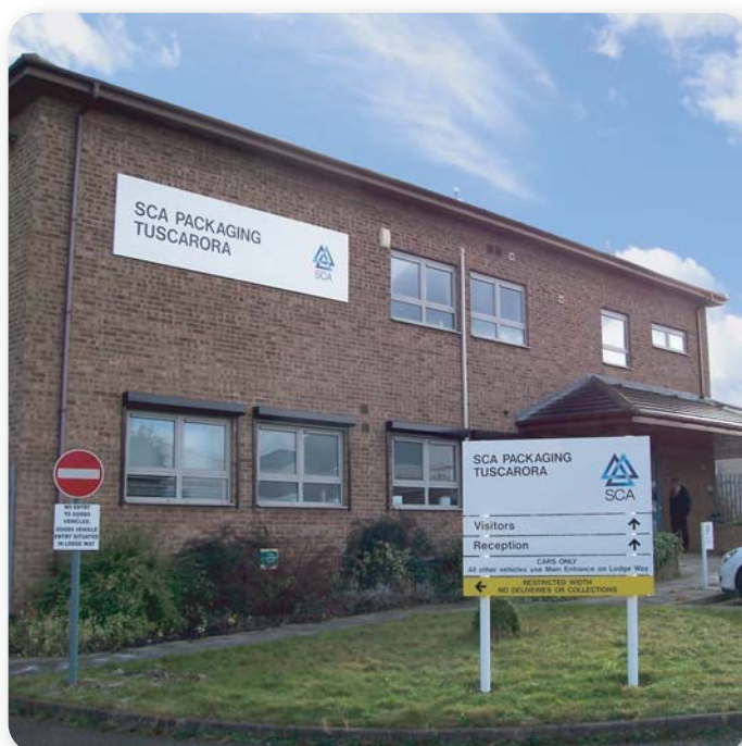
Building tray sign, directional post sign and traffic management sign
