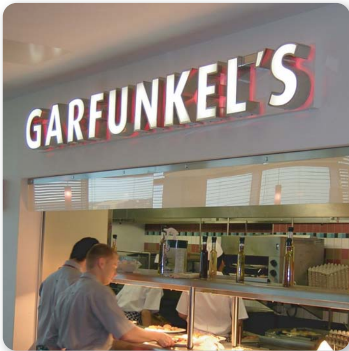
Internally illuminated built-up letters stood off bulkhead to give red halo
